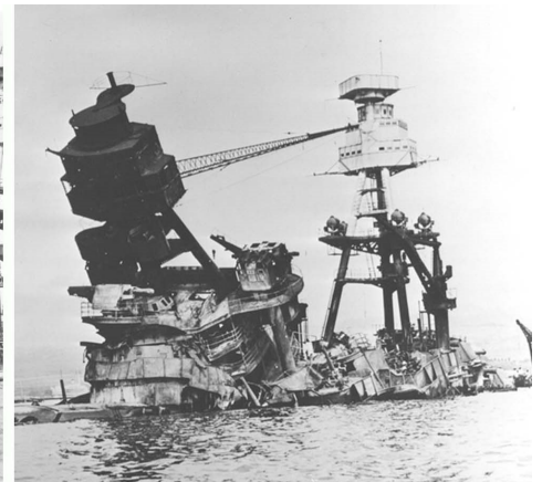
After fire has been extinguished (DEC 10, 1941)
