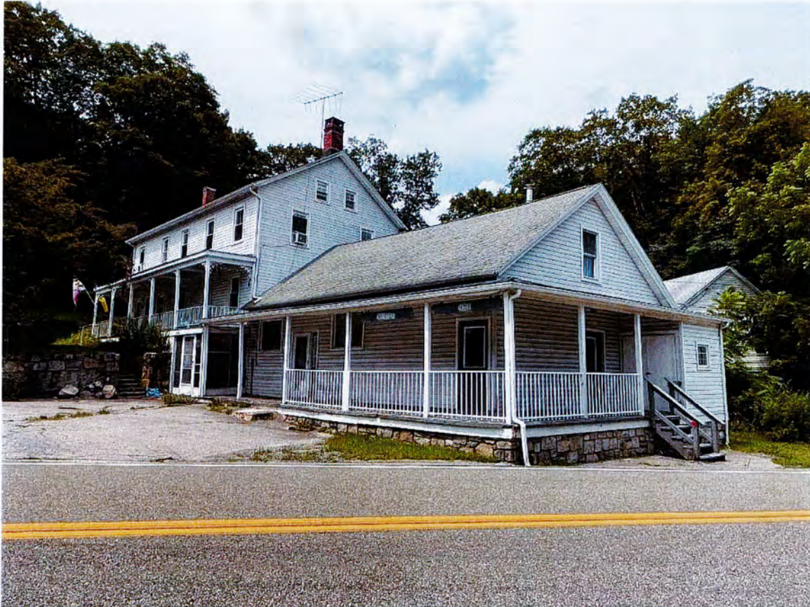
Photo 2. Structure 2, 721 Peekskill Hollow Road, looking north. Built c. 1875, this is a two-story, side-gabled, wood-frame single-family dwelling. Resting on a stone foundation, it is sheathed with novelty siding and it has an asphalt shingle roof. Fenestration is varied, consisting of replacement one-over-one, two-over-two, six-over-six and double hung sash. Projecting from the southeast elevation is a one-story, gable-roofed wing. The dwelling is not eligible for inclusion in the National Register of Historic Places due to loss of integrity resulting from alterations in the form of replacement windows and siding.
