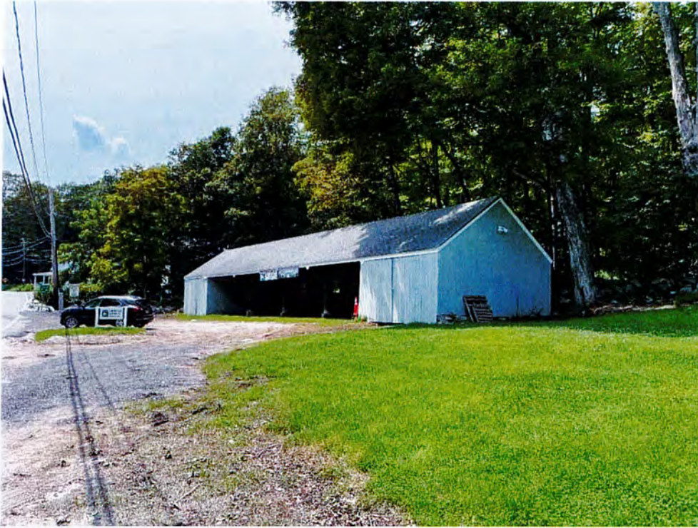
Photo 3. View looking west towards the extant carriage barn associated with the former Methodist church at 729 Peekskill Hollow Road.
