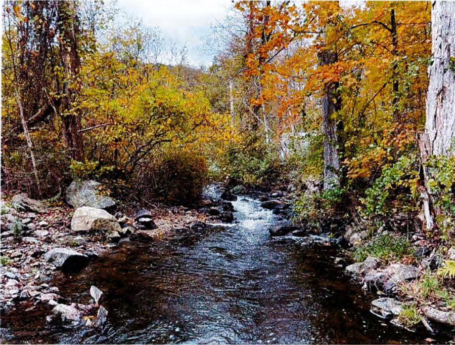
Photo 7: Looking upstream toward culvert.
