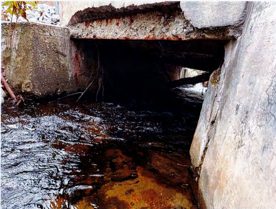
Photo 6: Looking northwest under the existing culvert.
