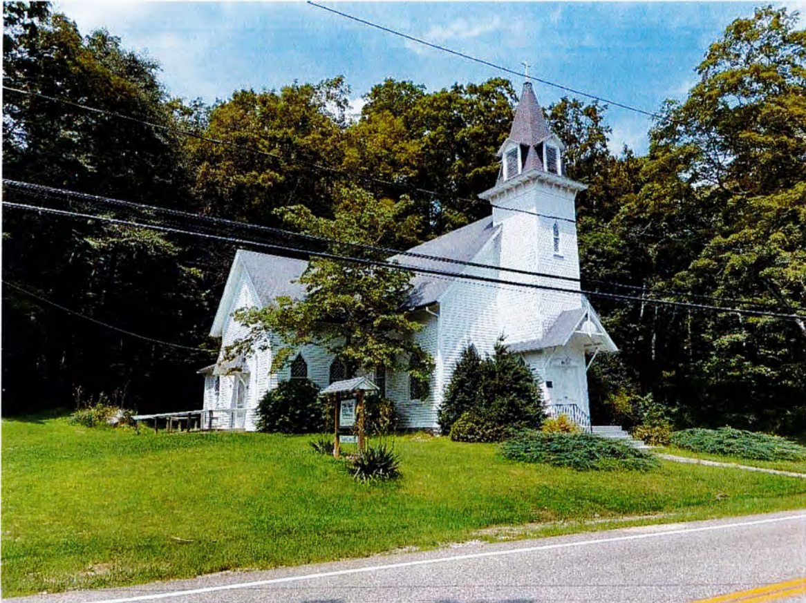
Photo 5. Structure 3, 729 Peekskill Hollow Road, looking north. Built in 1891, the National Register Listed Tompkins Corners United Methodist Church is an L-shaped, two-bay by-four bay, wood-frame religious building. Resting on a stone foundation, it is sheathed with wood clapboards, and it has an asphalt shingle roof. Fenestration consists of double-hung sash windows set with diamond-pane-stained glass. Projecting from the east elevation is a bell tower sheathed with sided with a mix of round, hollow-round, and diamond-shaped wood shingles. The tower is capped by a pyramidal roof with gable-roof dormers and a bracketed cornice. The Tompkins Corners United Methodist was listed on the National Register in October 1982 and retains integrity of location, design, materials, workmanship, feeling and association.
