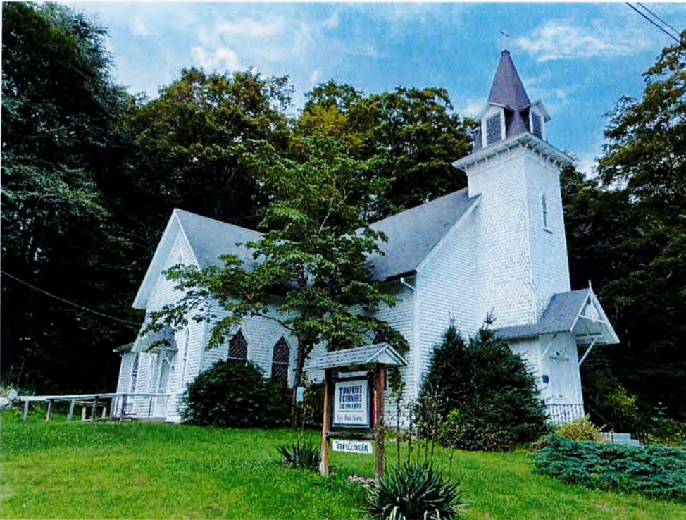
Photo 1. View looking north towards the NR Tomkins Corners United Methodist Church (90NR02380), presently known as the Tomkins Corners Cultural Center. While this structure is situated outside of the APE, the APE intersects the southern portion of the property.
