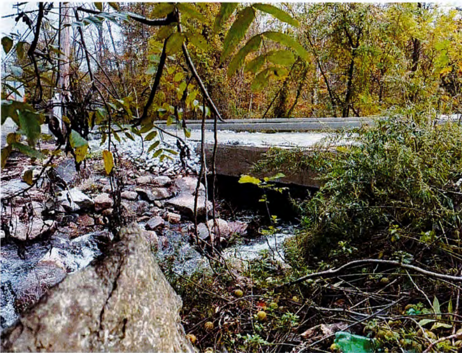
Photo 4: View of culvert looking southeast.
