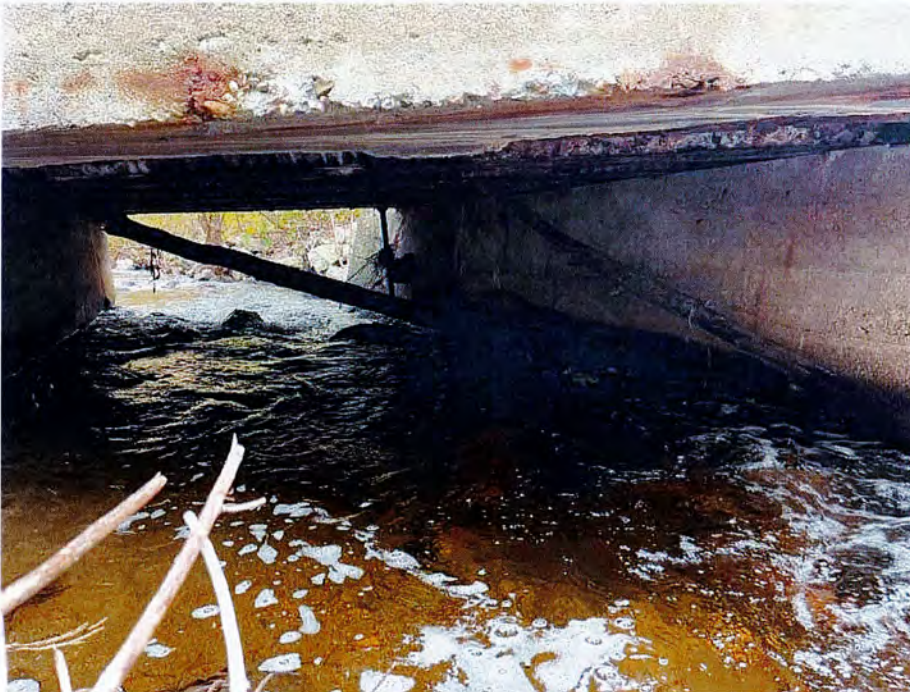
Photo 8: View looking west under the culvert.
