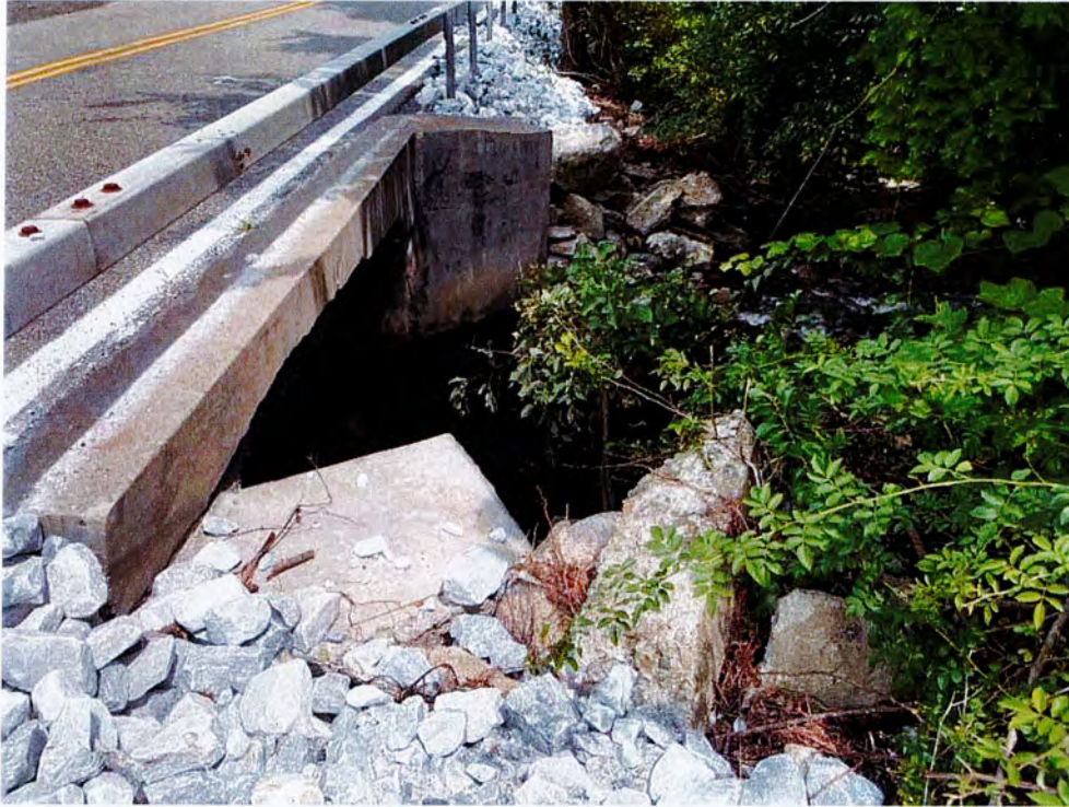
Photo 11. View looking northeast towards the eastern side of the culvert.
