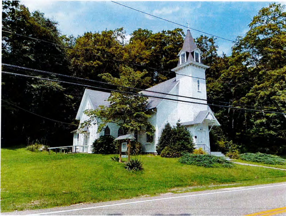
Photo 1. View looking north at the National Register Listed (NRL) Tompkins Corners United Methodist Church at 723 Peekskill Hollow Road.
