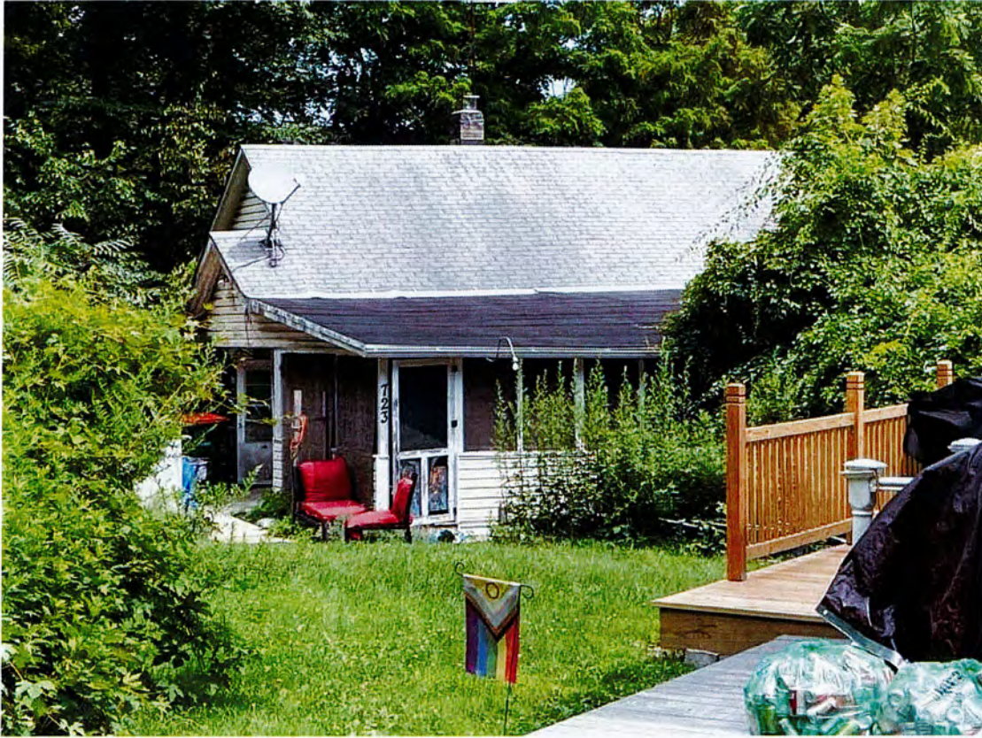
Photo 3. Structure 2a, 723 Peekskill Hollow Road, looking east. Built c.1940, this is a one-story, gable-roofed, wood-frame single-family dwelling. Resting on a concrete block foundation, it is sheathed with novelty siding and it has an asphalt shingle roof. Fenestration consists of six-over-one replacement windows. A one-story, hip-roofed enclosed porch extends along the south elevation. The east elevation is exposed at the basement level with a built-in garage. The structure is not eligible for inclusion in the National Register of Historic Places due to loss of integrity resulting from alterations in the form of replacement siding and windows.
