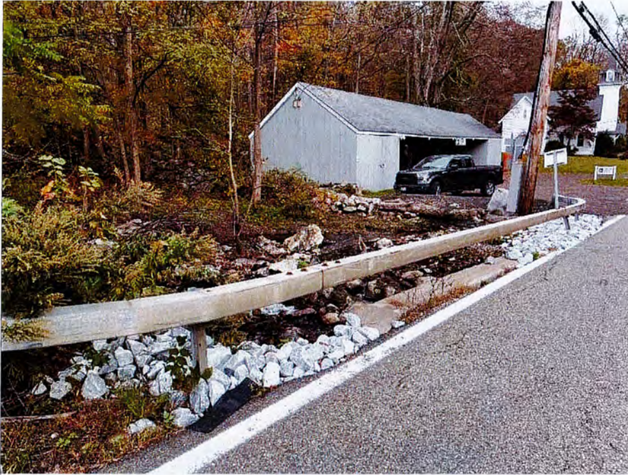
Photo 3: View of culvert looking northeast.
