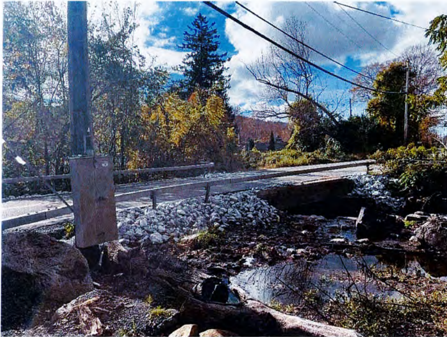
Photo 1: View of existing culvert looking southwest.
