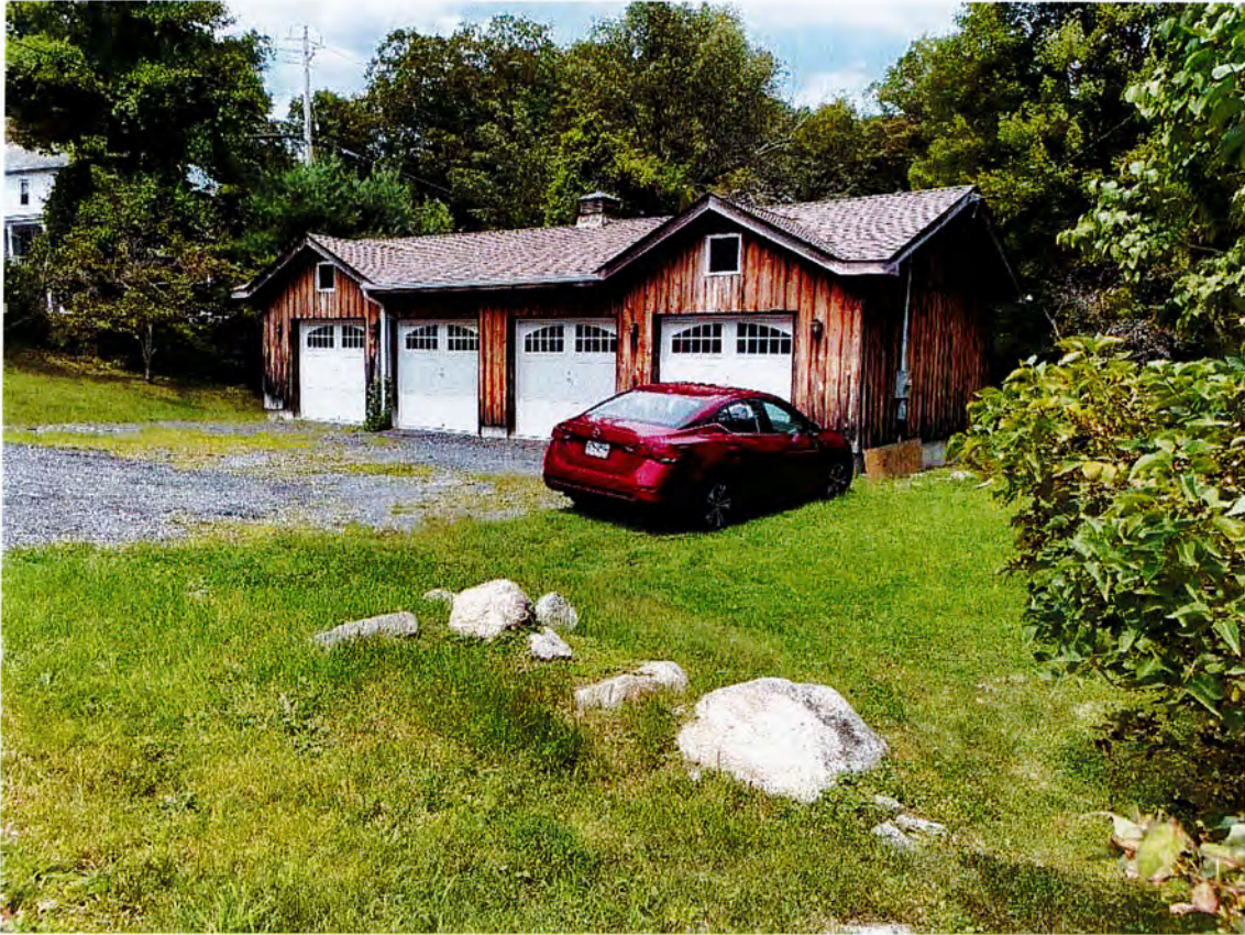
Photo 4. Structure 2b, 721 Peekskill Hollow Road, looking north. Built c.2005, this is a one-story, four-bay, side-gabled garage. Resting on a concrete slab, it is sheathed with vertical wood boards and it has an asphalt shingle roof. The structure is not eligible for inclusion in the National Register of Historic Places due to insufficient age.
