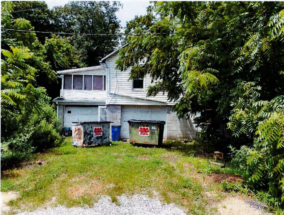
Photo 4. View looking northwest towards the structure at 723 Peekskill Hollow Road.
