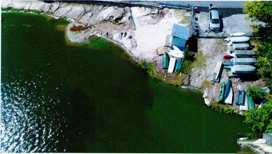
Lake Peekskill Culvert replacement project. Summer 2024. Part 'C' Funded.
